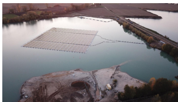
Fig. 5.7: Example of floating PV (1.5 MW electric peak power) plant in Leimersheim near the Rhine
